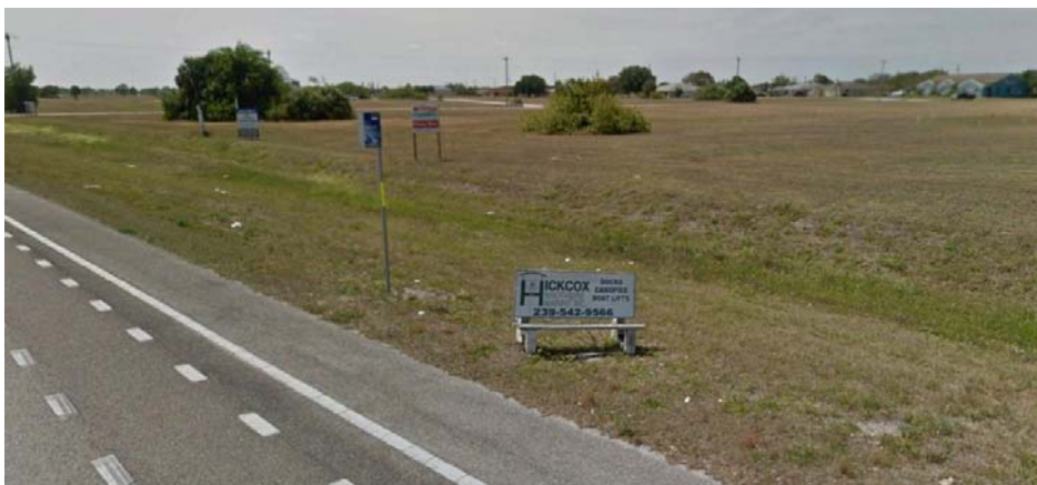
Existing Bus Stop along North Side of SR 78 (No sidewalk connection with sign and bench located within Open Swale area)
